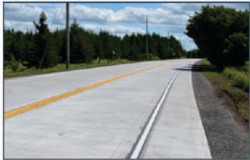
Wide Concrete Road
