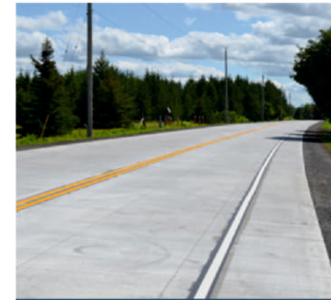
Internal Cement Concrete Road
